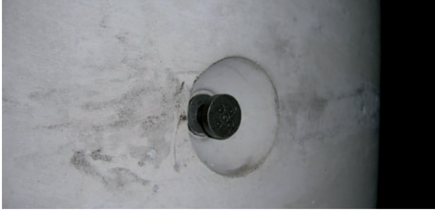
Cast in lifting anchors for safe product handling on the building site.
