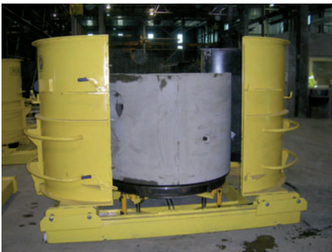
The cured monolithic monobase is ready for de-moulding.
