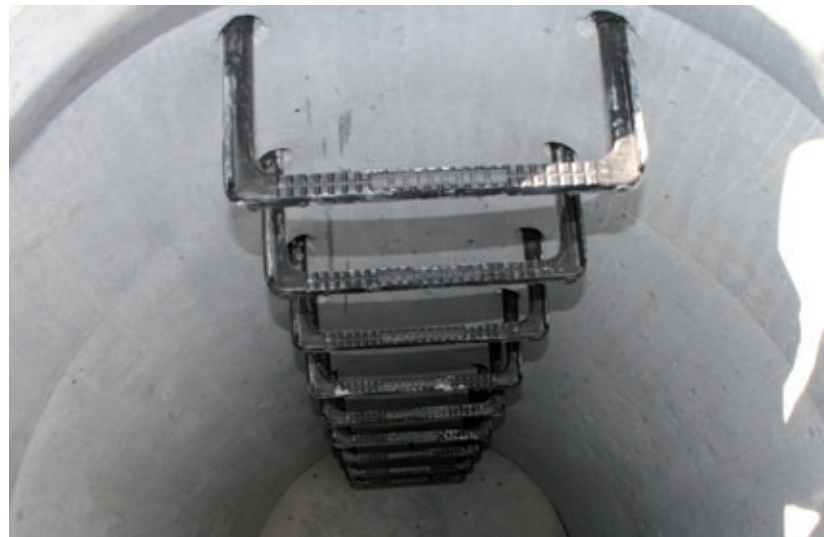
After de-moulding, the steps are knocked into in designated bushings
