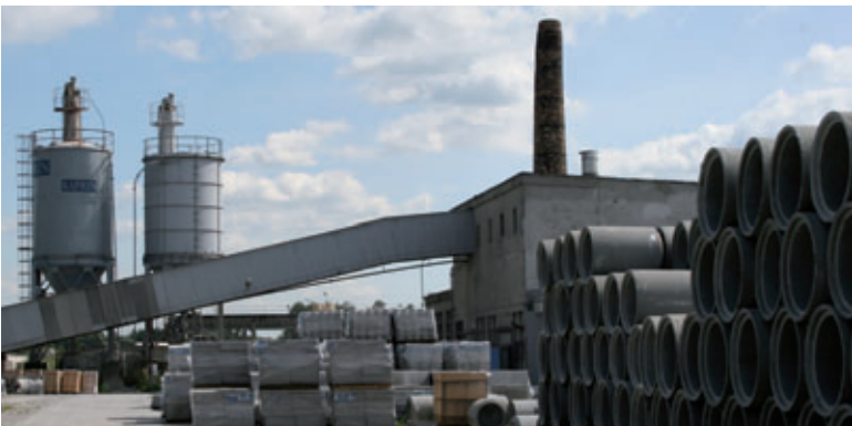
The Kaprin Sp.z o.o. plant in Krzeszowice
