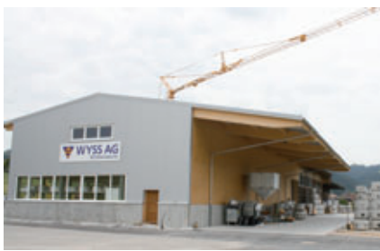
This newly erected hall extension is where O. Wyss AG produces monolithic perfect manhole bases
