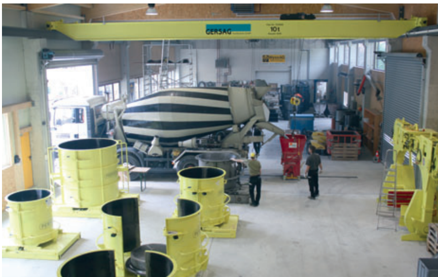
The mixer trucks drive backwards into the hall and the concrete is transferred into a concrete bucket
