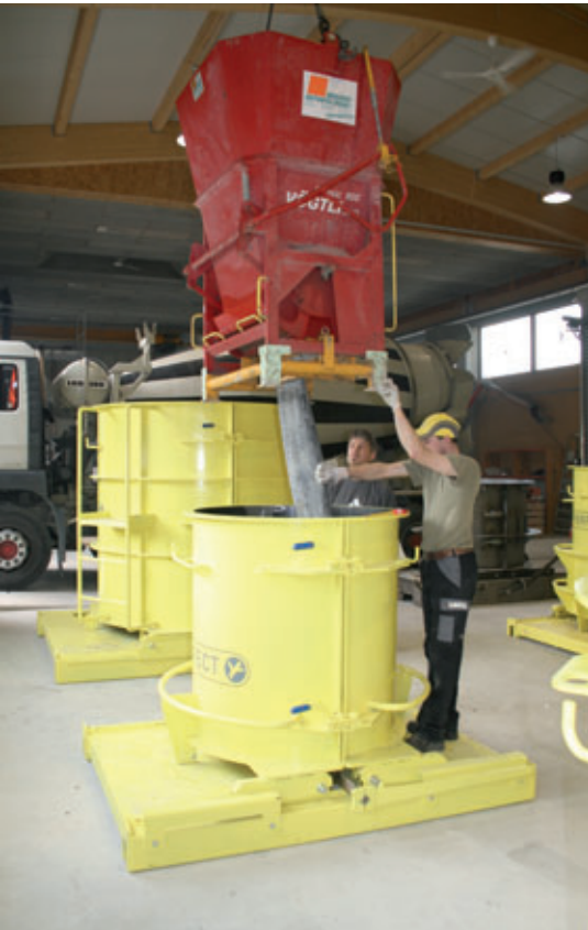
Concreting is done with a concrete bucket
