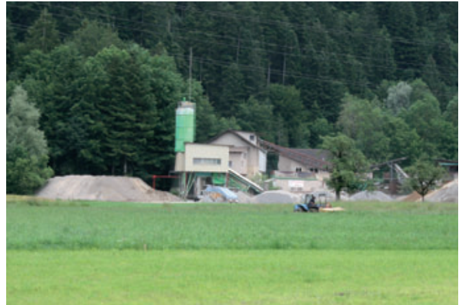
The concrete is delivered from the ready-mix plant just a stone's throw away
