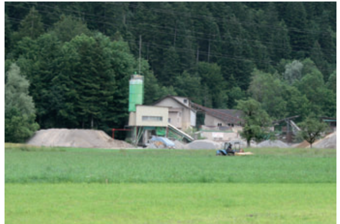
The concrete is delivered from the ready-mix plant just a stone's throw away
