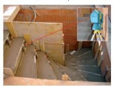
rings. On a portable tripod about 360 degrees swivelling stored ProCollector and the wireless service unity ProCommander are used on building sites as a time-saving dimension system of the stair construction, casings and the inside removal.
