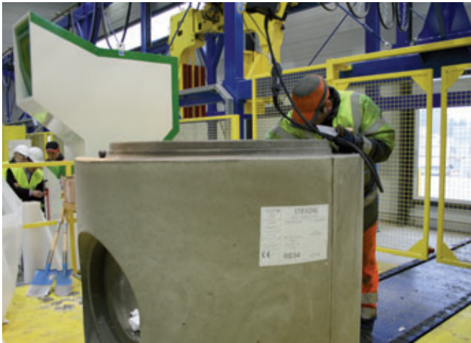
Removal and recycling of the recess units
