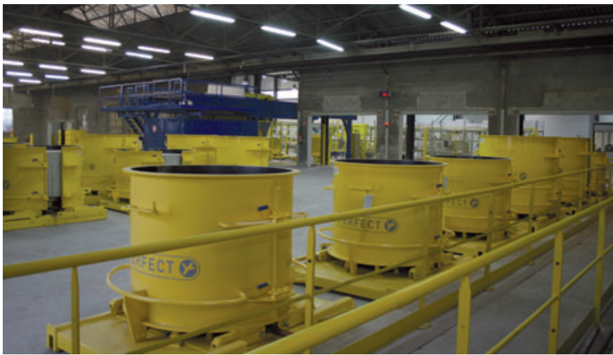
The freshly filled moulds are brought to the storage area in tipper trucks
