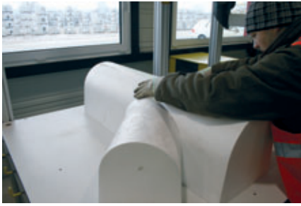
The individual cut sections are put together, the channel courses shown by a laser projection help to correctly position the moulded parts
