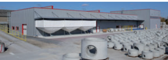
At the Kilstett plant Stradal recently launched the second Perfect manhole base production by Schlüsselbauer
