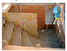
360 degrees swivelling stored ProCollector and the wireless service unity ProCommander are used on building sites as a time-saving dimension system of the stair construction, casings and the inside removal.
