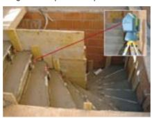
degrees swivelling stored ProCollector and the wireless service unity ProCommander are used on building sites as a time-saving dimension system of the stair construction, casings and the inside removal.
