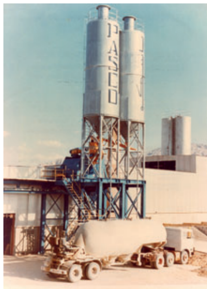
Pasco No. 1 with Mixing Plant
