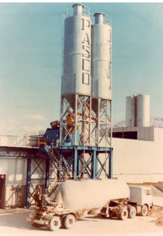
Pasco No. 1 with Mixing Plant
