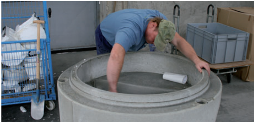
Removal of the recess units
