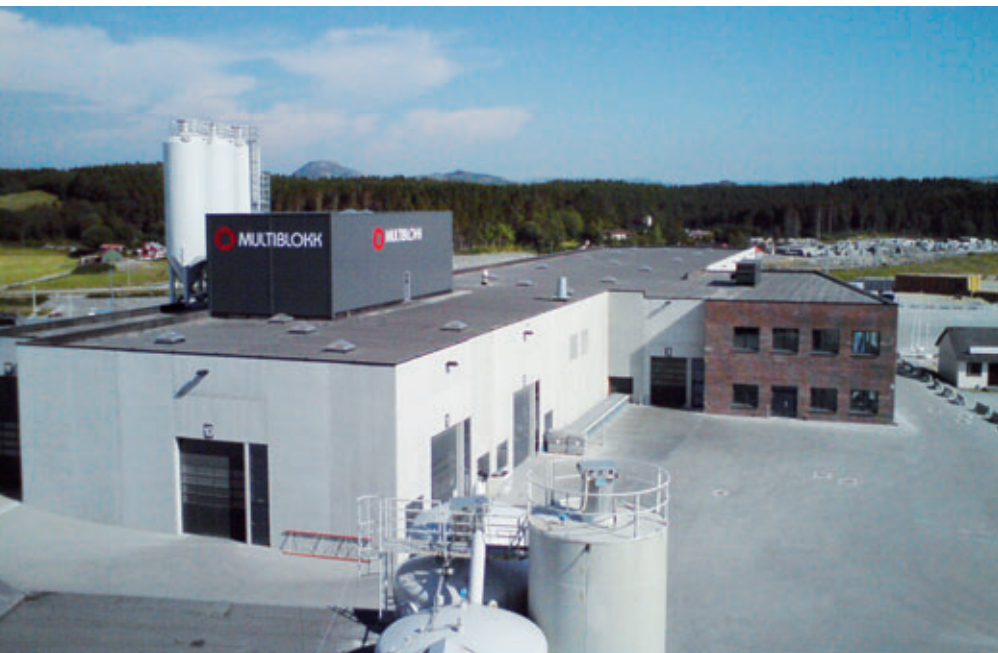
The Multiblokk site in Sandnes, Norway
