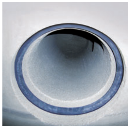
All seals for the connections are glued in place with a polymer adhesive in the recess provided
