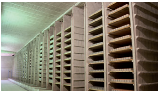
The rack unit consists of 31 chambers with a capacity of 10,200 boards
