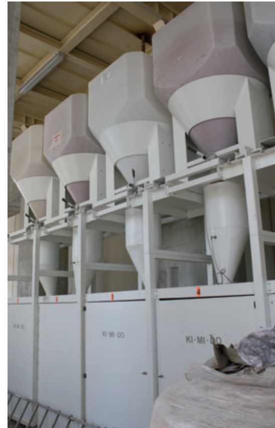
The dye dosing equipment by the German company Kimido Kindler GmbH
