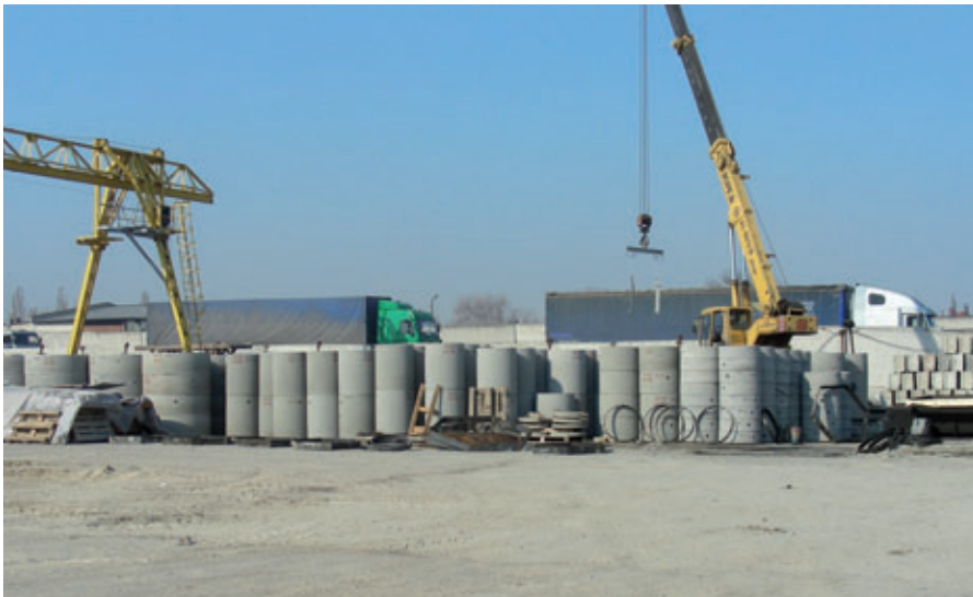
Manhole elements in the loading area at OOO <<SMK-50>>
