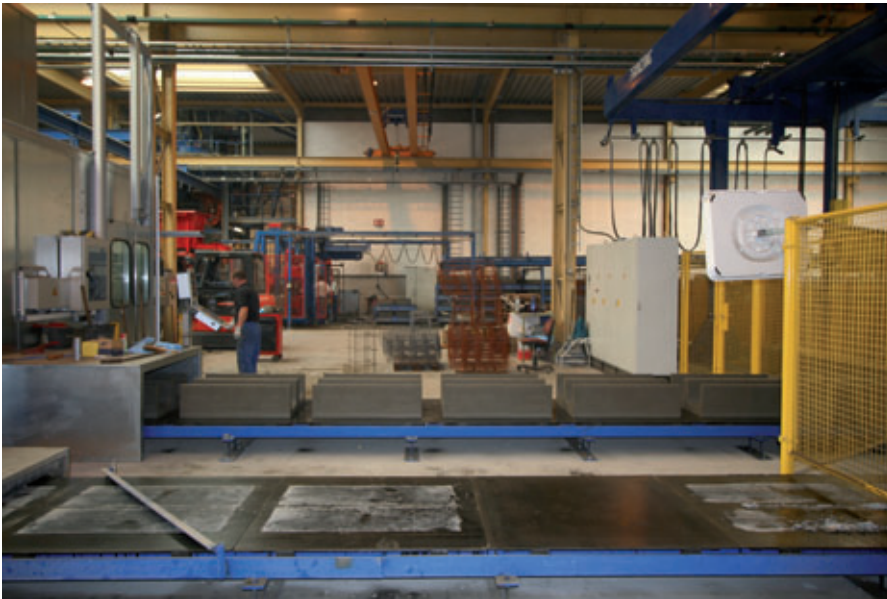
Background: fresh concrete products being transported from production to the warehouse. Foreground: empty pallets being returned to the production circuit via the automated pallet cleaning machine
