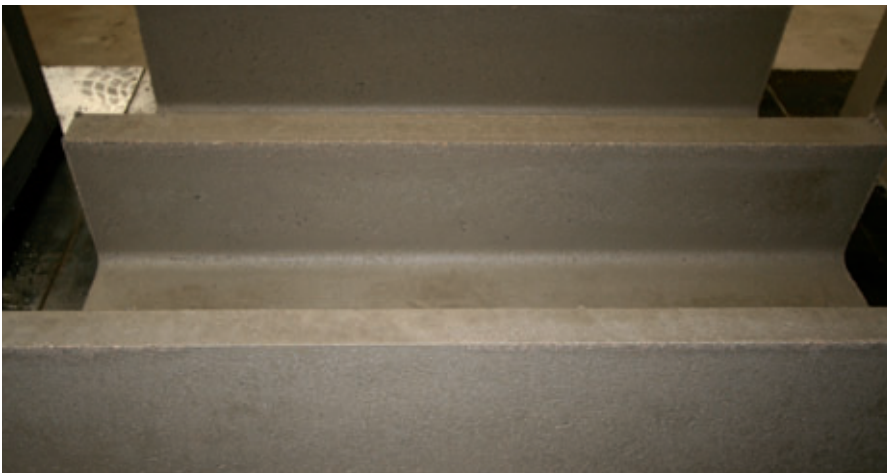
Impressive external appearance of the Roeselare cable ducts
