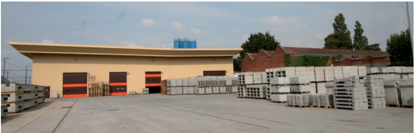
The Infrabel concrete production facility in Roeselare featuring the latest equipment
