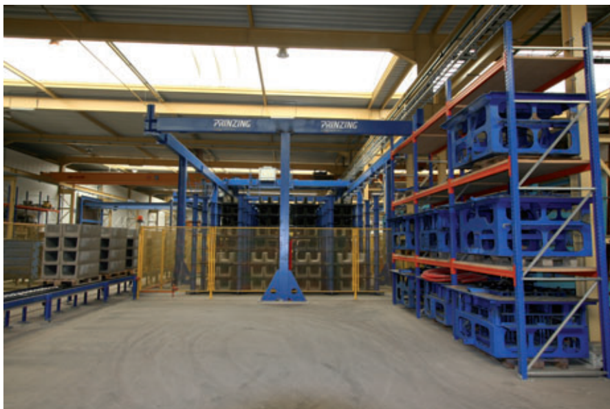
At Roeselare, the plant was designed to allow the curing rack to be enlarged to cater for possible two-shift operation
