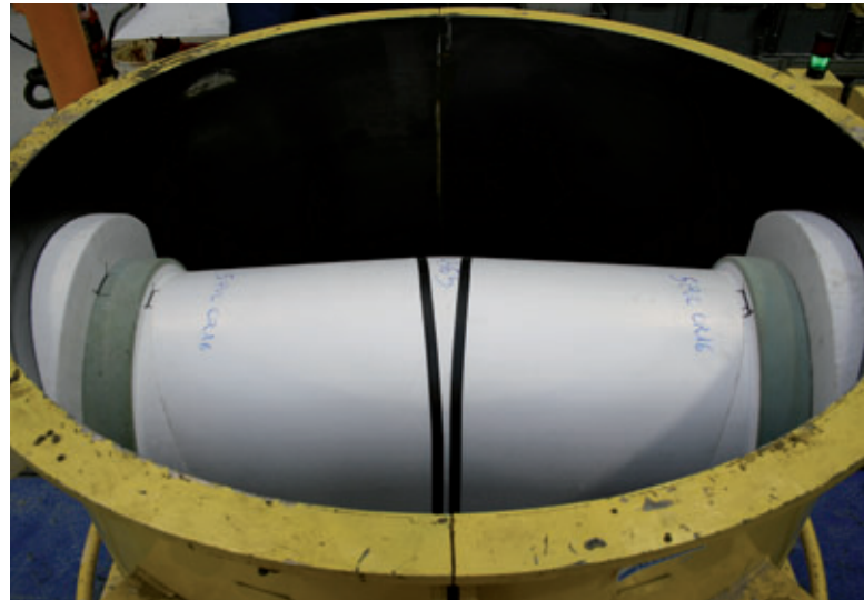
A steel mould complete with a negative channel piece is ready to be poured with self compacting concrete (SVB).
