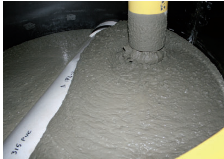
The filling of a mould with self compacting concrete C40/50.
