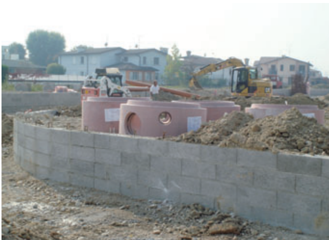
Application of high quality concrete manhole bases produced by the company Buzzella Ennio SRL
