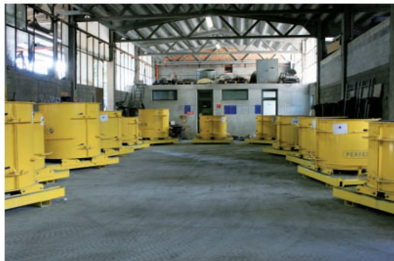
View of the production building at Buzzella Ennio SRL: Perfect moulds for the production of manhole bases DN 1000 and DN 1200.
