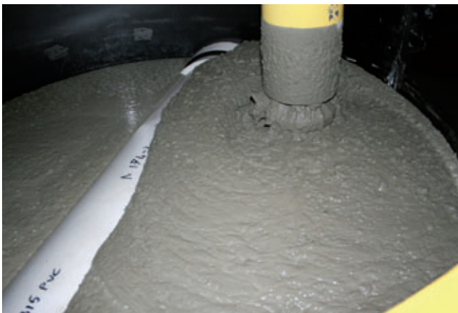
The filling of a mould with self compacting concrete C40/50.
