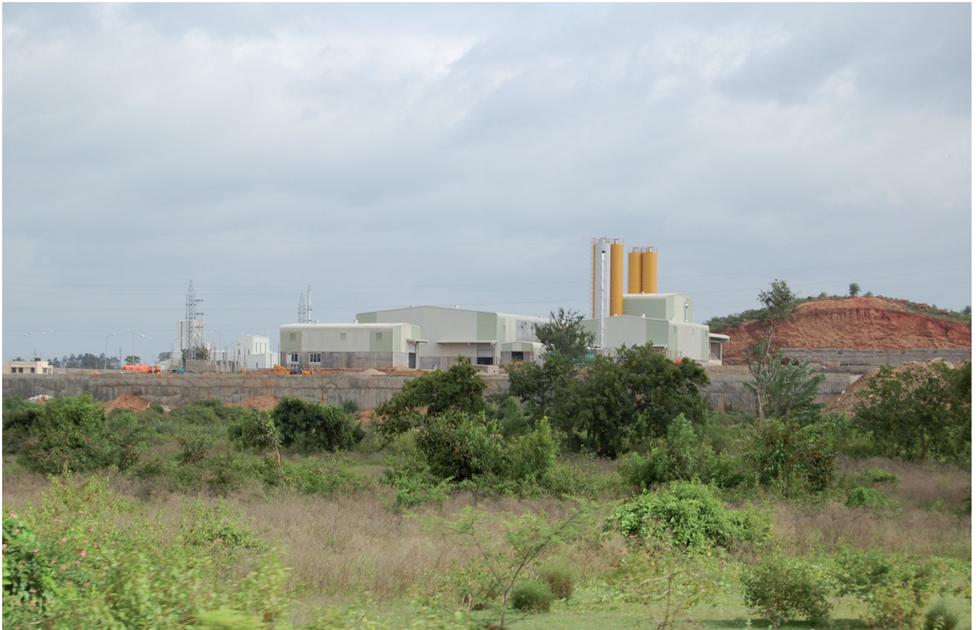
Building ground for Basant Betons
