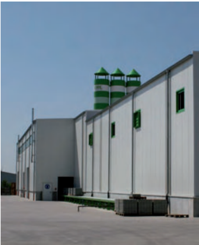
The new EHL concrete plant in Ahlhorn
