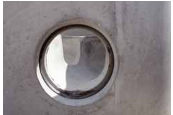
Pipe connection with a joint gasket
