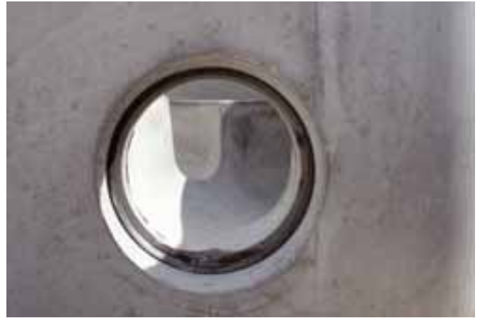
Pipe connection with a joint gasket
