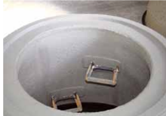
Insertion of the step rungs is an easy job using the Stepmaster
