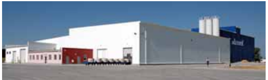
The brand-new facility of ZPB Kaczmarek at Prusice – in the front the out feed conveyor of the manufacturing system „Perfect“
