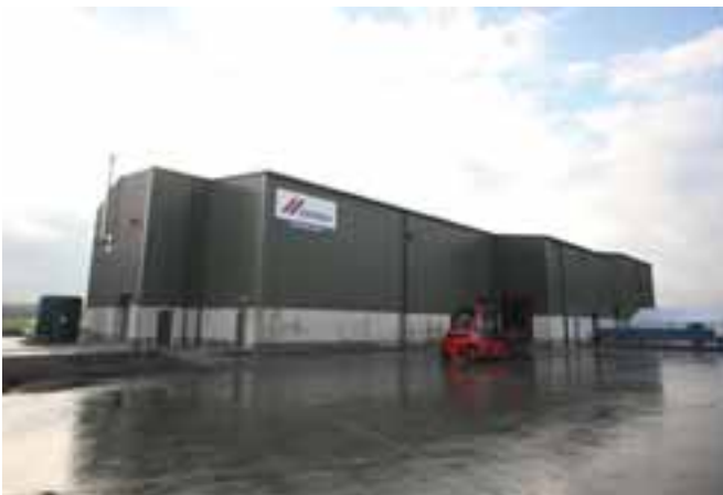
The new concrete block and paving plant in Scotland
