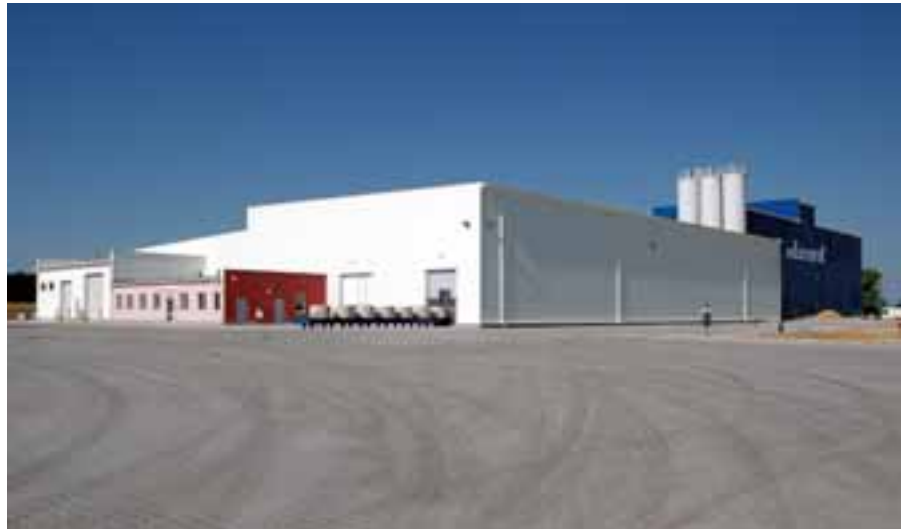
The brand-new facility of ZPB Kaczmarek at Prusice – in the front the out feed conveyor of the manufacturing system „Perfect“
