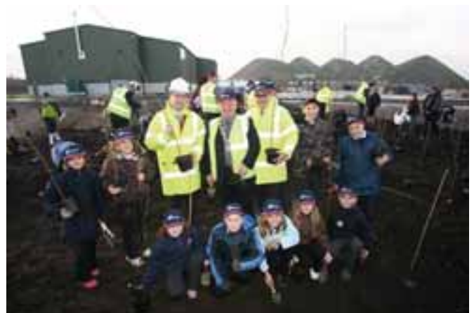
Children from nearby St Mary's Primary School helped mark the occasion by planting 100 trees, as part of Cemex's commitment to sustainable development
