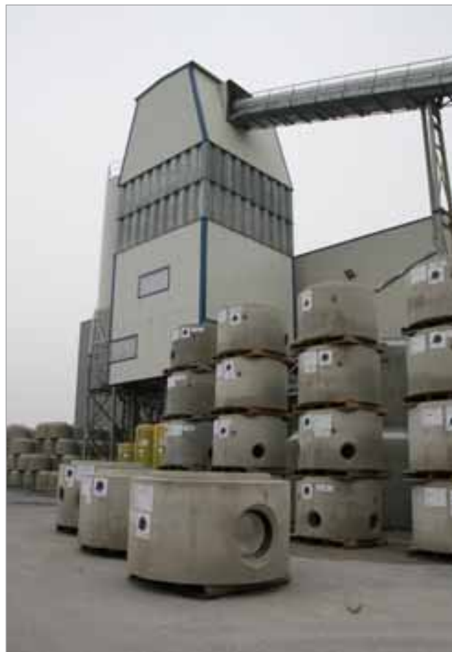
In order to be self-sustaining each hall at Plattard disposes of an own mixer for concrete.
