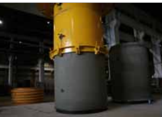
Outfeed of the filled mould out of the pipe station and its transfer to dismantling.
